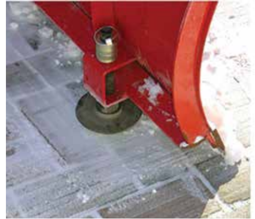
Figure 5. Shoes on plows need to be adjusted so the blade is not pushed across the surface and limits scratching the pavers.
