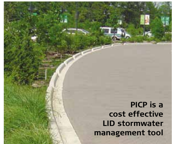
PICP and bioswales work together as LID tools to increase infiltration at Morton Arboretum in Lisle, IL.
