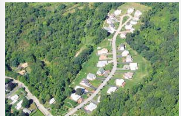
By eliminating detention pond, the subdivision layout conserves trees while 15,000 sf (1500 m 2 ) PICP in the cul-de-sac returns rainfall to the water table in Glen Brook Green subdivision in Waterford, CT.
