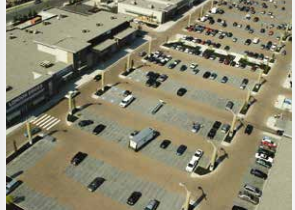
350,000 sf (3.2 ha) of PICP at a Burnaby, BC shopping center infiltrates runoff from roofs.
