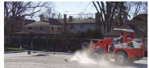
Mechanical sweeping of fine aggregate into paver joints
