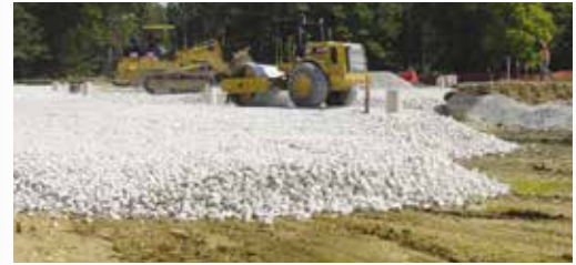
Base construction uses locally available materials.
