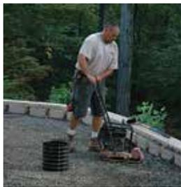
**Compaction:** Once the soil type is identified, the contractor needs to compact it. Compaction achieves four main purposes: it increases the soil's load-bearing strength; prevents pavement settlement/rutting; reduces seasonal movement; helps ensure that any movement is uniform. When compacted properly, the aggregate base density will minimize deformation and/or heaving of
