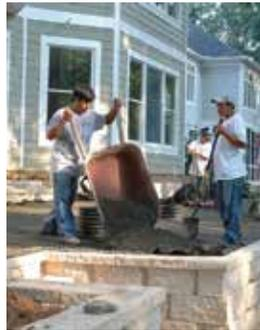
**Soil type:** A properly prepared soil subgrade supports the base above it and distributes the loads from the surface. The soil type should be identified before starting the job, during the bid proposal. It can affect the estimate on labor hours and the type of equipment required for the job.
