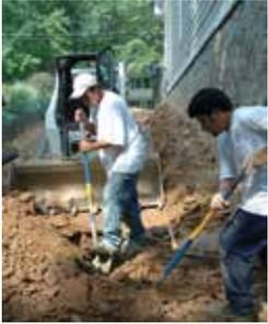
**Site layout and excavation:** The layout of interlocking concrete pavement translates the drawing into reality. In addition to knowing the size of the pavement and excavated area, the layout tells the contractor the sequence of job functions and crew involvement. Considering all factors in advance such as material storage and paving direction helps ensure a smooth operation.
