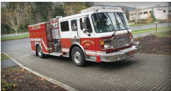
This PICP fire station driveway in Snoqualmie, WA eliminates runoff during most rainstorms.
