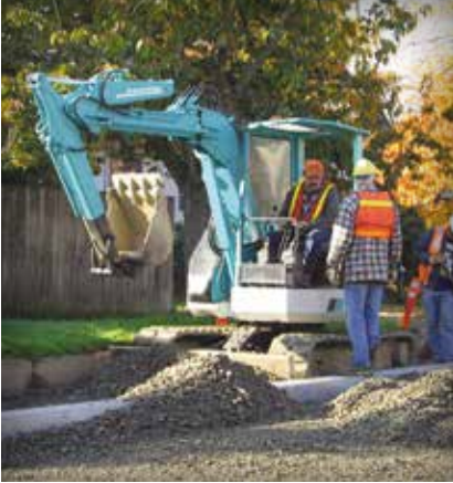
Prepared subgrade for 20,000 sf (2000 m 2 ) Portland, OR street retrofit with PICP
