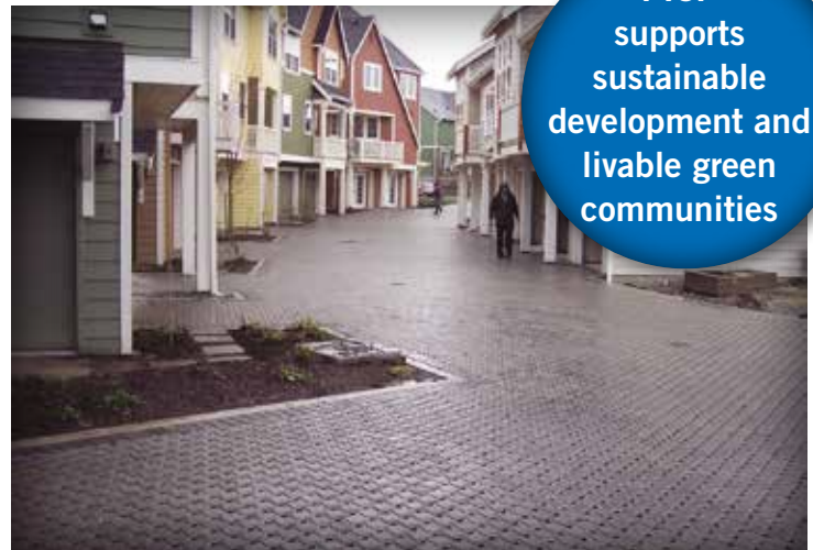
PICP's can eliminate street storm drains and sewer pipes as in this redevelopment project in Seattle, WA.
