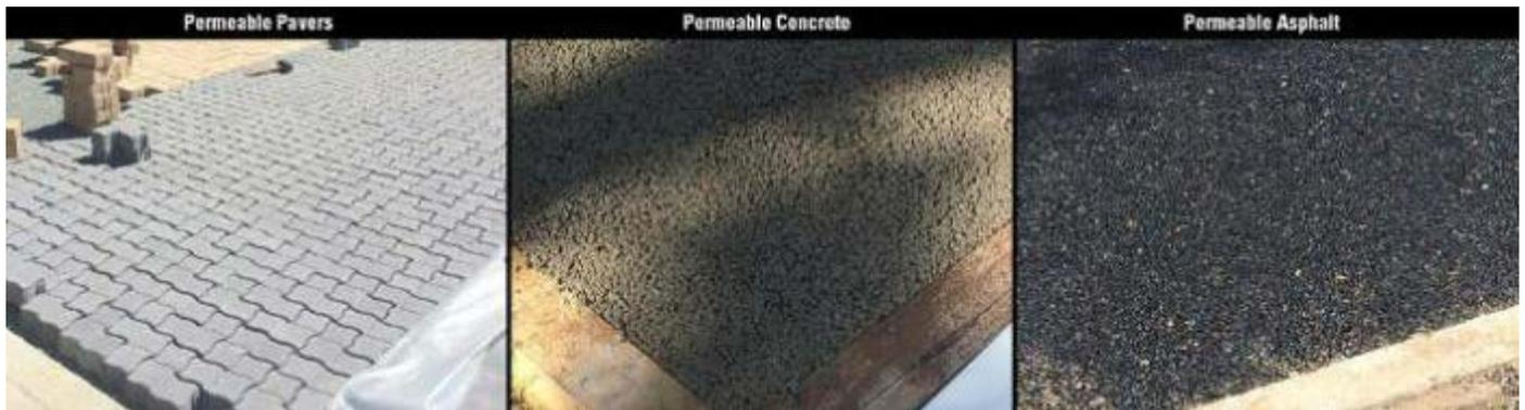
Permeable pavement is a porous urban surface which catches precipitation and surface runoff, storing it in the reservoir while slowly allowing it to infiltrate into the soil below. This study will evaluate how well different types of permeable pavement reduces the amount of pollutants and runoff volume. [More.](#)
