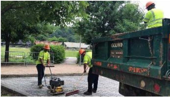
"These are permeable pavers that allow for water to soak through the pavers, go into the ground. It filters out a lot of the pollutants that we have in the water from cars and vehicles and things like that and then it discharges into the James River," said Jes Gearing with the Lynchburg department of Water Resources. [More.](#)
