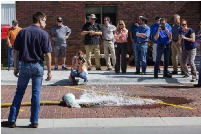
A blast from a fire hose Wednesday morning showed how stormwater will now — instead of running straight into a storm drain — seep into cracks between the new brick pavers that line a block in this Johnson County city's downtown.
