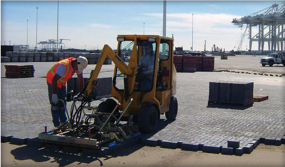
Figure 8. Mechanical installation equipment places concrete pavers rapidly.
