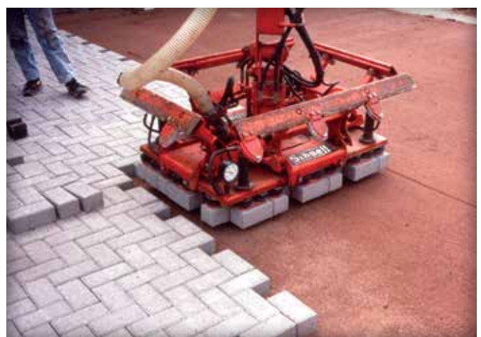
Figure 6. The vacuum head over the paver layer.
