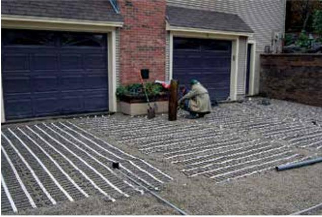
Figure 10. Electric heat tape snow melt system is installed in the bedding layer of permeable interlocking concrete pavement.
