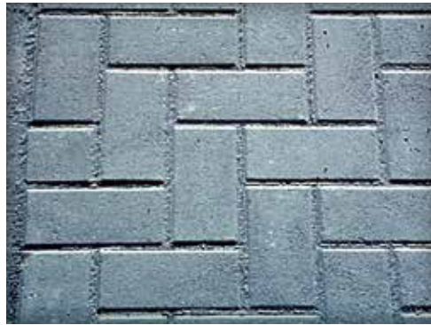
Figure 6. A close-up of the concrete paver surface at the PTI test track.
