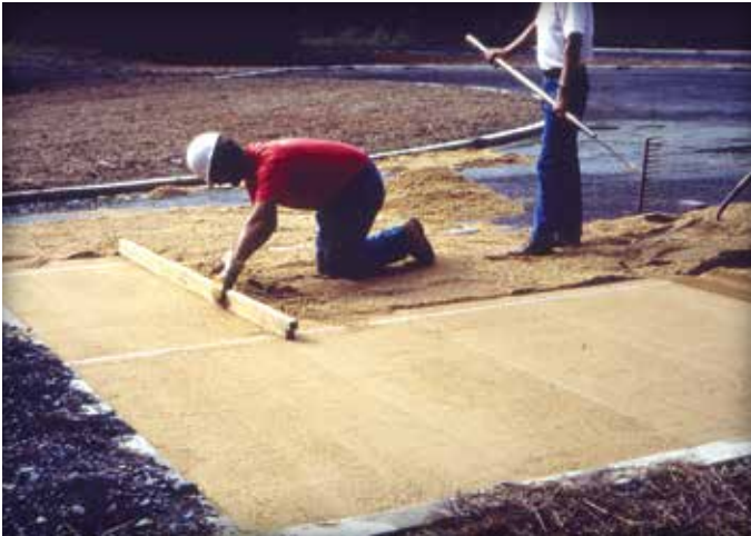
Figure 6a & 6b. Screeding the bedding sand.
