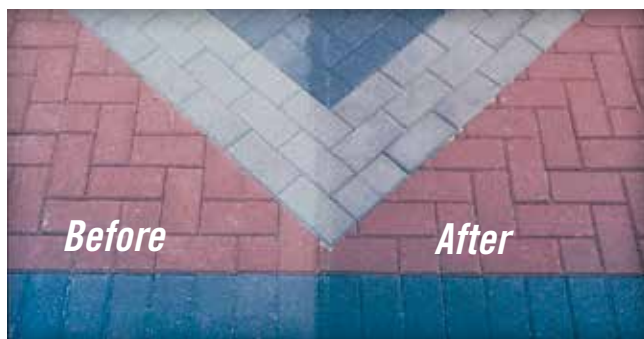
Figure 8. Before and after application of an acrylic sealer shows how it deepens the appearance of concrete pavers.
