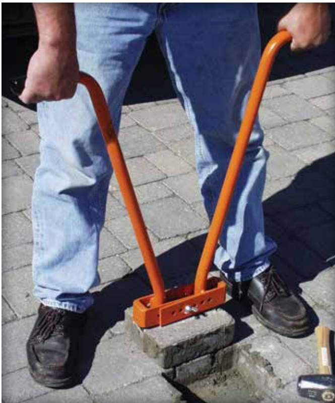
Figure 5. Using a paver extractor to remove a paver
