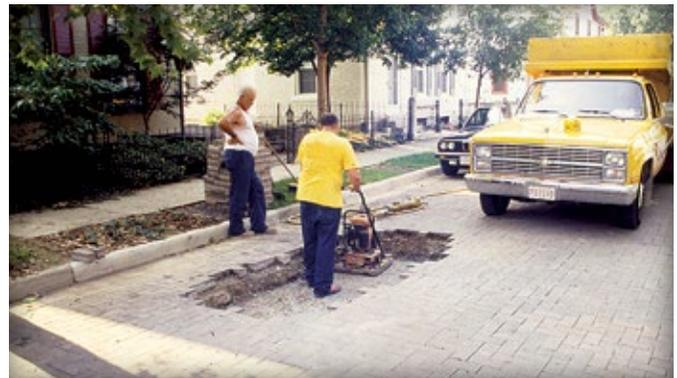
Figure 3. Compaction of the base
