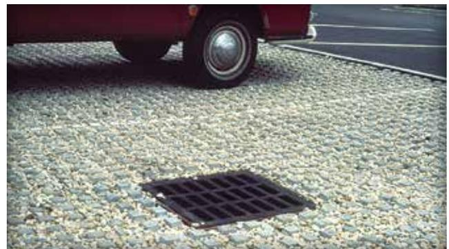
Figure 16. Concrete grids with aggregate in the openings
