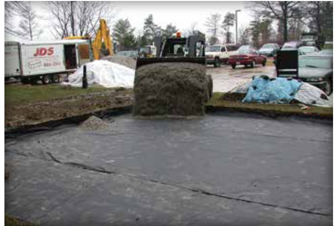
Figure 3. Application of the geotextile under aggregate base.
