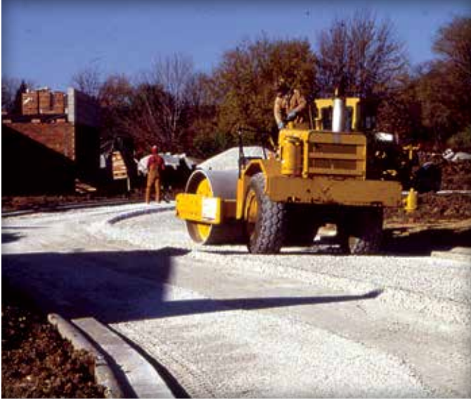
Figure 4. Base compaction with a vibratory roller.
