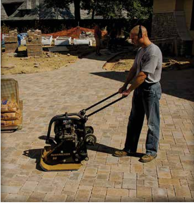
Figure 9. Compacting the pavers and bedding sand.
