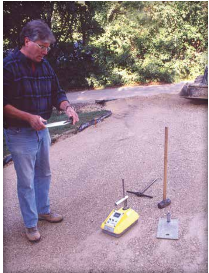
Figure 5. Density testing of the aggregate base with a nuclear density gauge.
