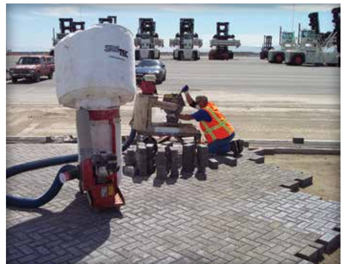
Figure 8. Saw cutting pavers.
