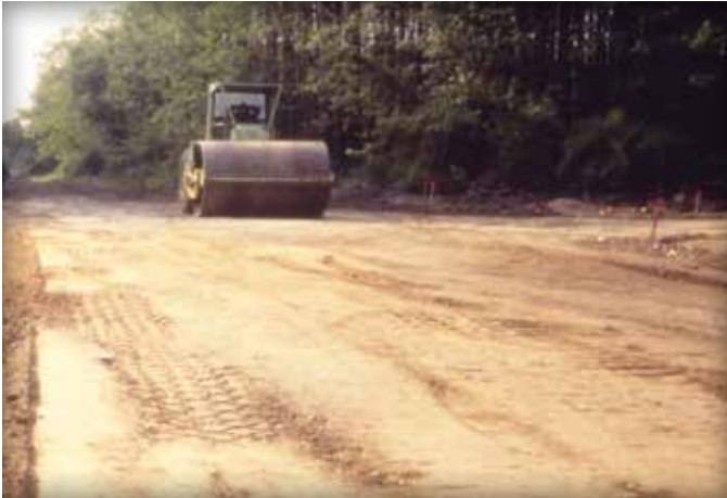
Figure 2. Compacting the soil subgrade.
