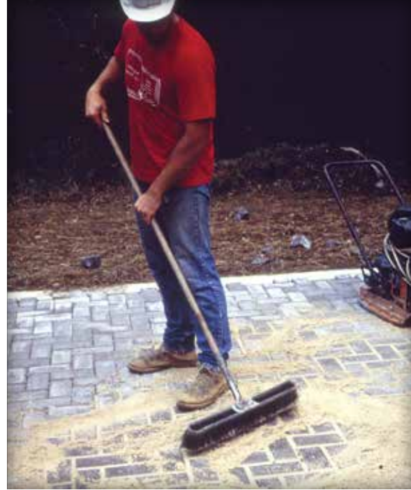
Figure 10. Spreading and sweeping joint sand.
