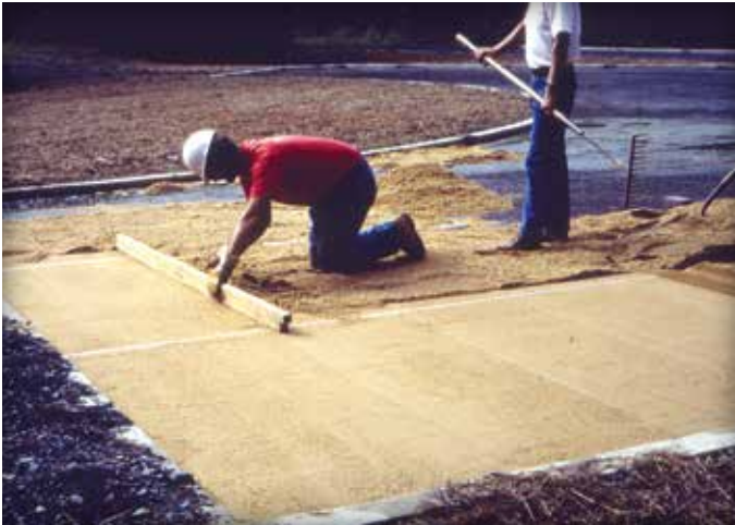
Figure 6a & 6b. Screeding the bedding sand.
