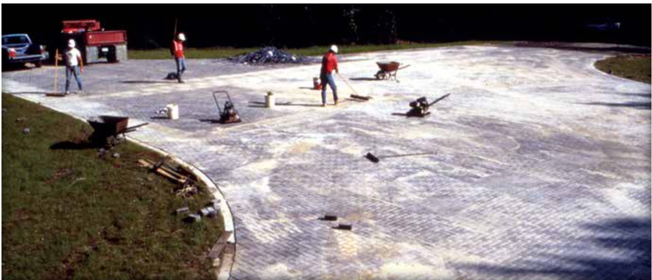
Figure 12. Excess sand swept from the finished surface will make the pavement ready for traffic.
