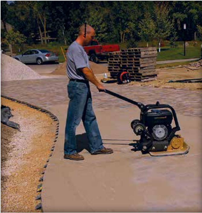
Figure 11. Vibrating sand into the joints.
