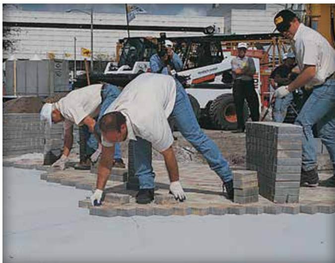
Figure 7. Placing the concrete pavers.
