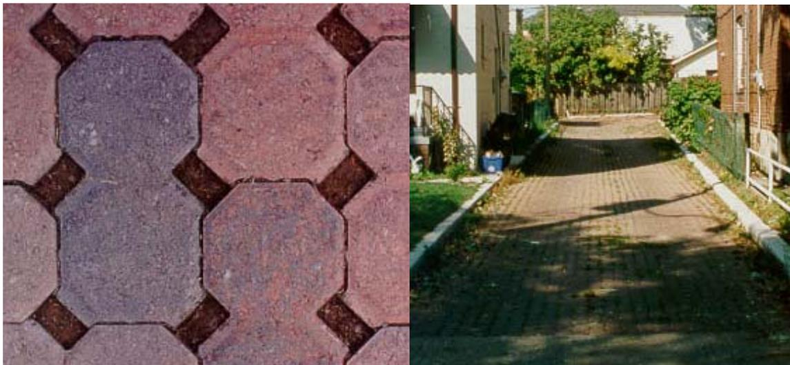
**Figures 1 and 2. UNI Eco-Stone permeable pavers and a typical application.**
