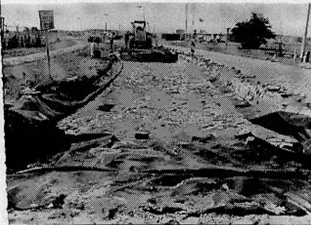
Figure 2 Overview during execution
