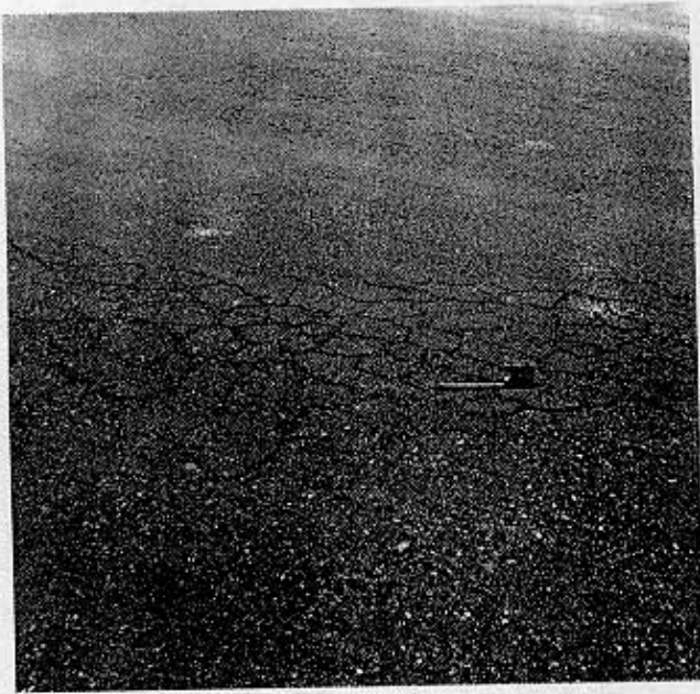
Figure 4. Cracking of rehabilitated asphalt surface at the access way to the junction.
