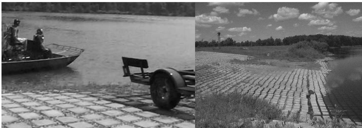
**Figure 2. Cable articulated mat made by attaching the blocks at four points to form a block paving for a landing ramp.**
