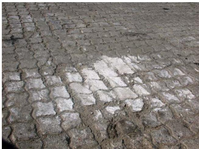
**Figure 11. Damage to CBP Pavement Caused by Tracked Equipment**
