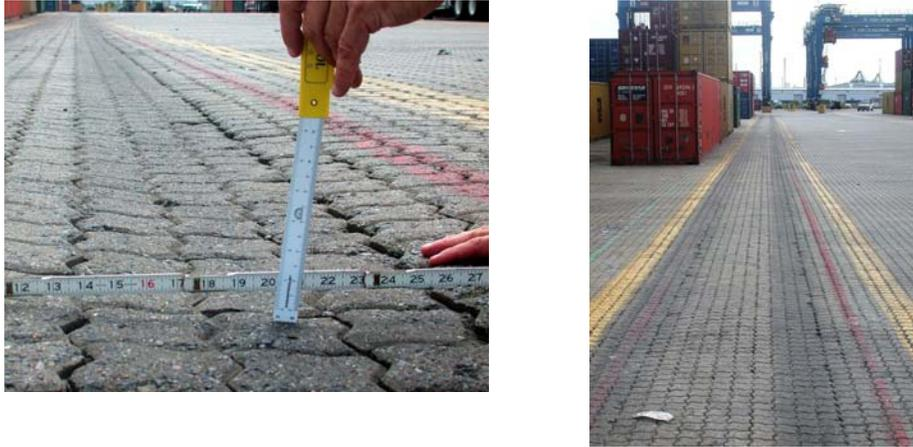
**Figure 8. Rutting from RTG Operation**
