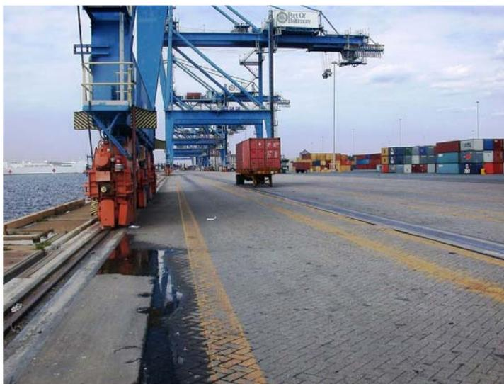
**Figure 5. CBP Pavement at Seagirt Berths 1, 2, 3**
