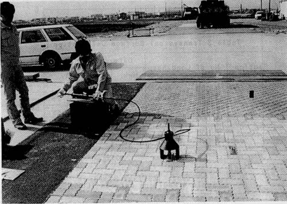
Photo 4 Direct Pulling Test
