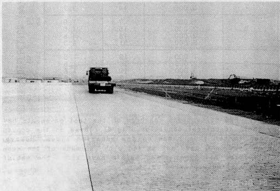
Photo 3 Repetitive Loading Test
