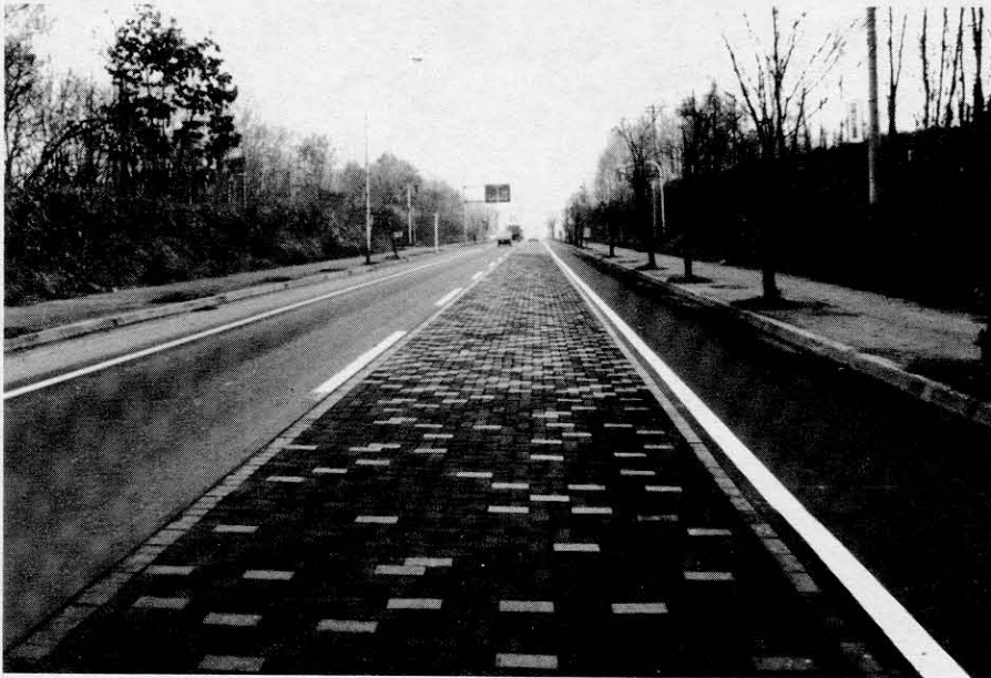
Fig. 8 - ASSEC application to street paving
