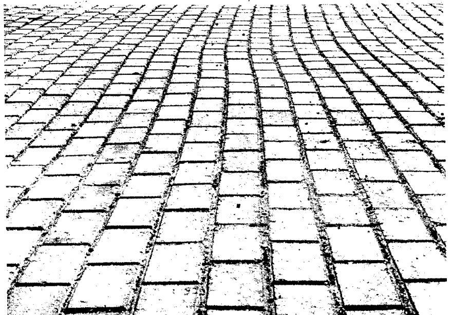
Figure 4: An example of "creep" in blocks laid in a stretcher bond pattern.
