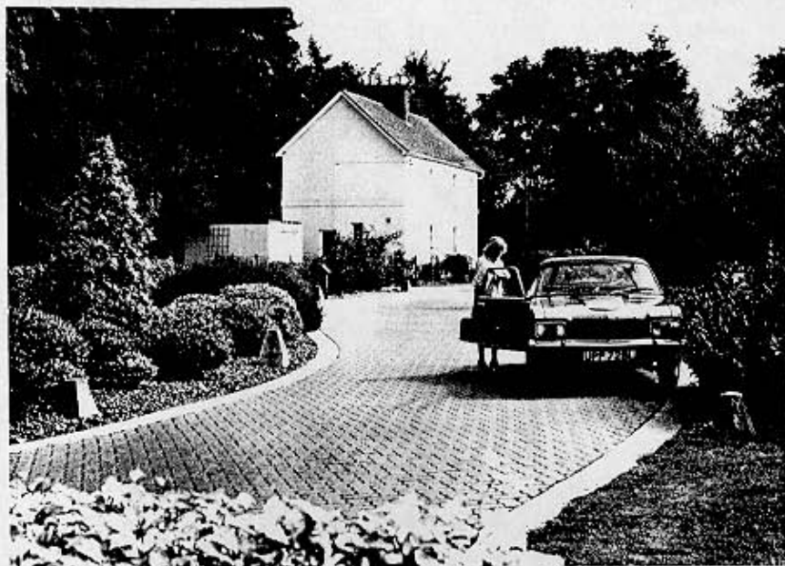
Figure 1: A five-year old block road on a 75 mm concrete sub-base.
