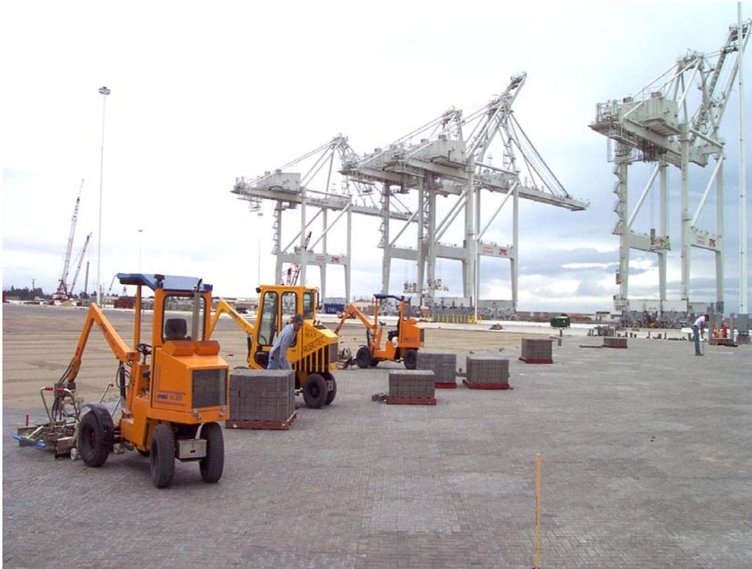
**Figure 5. Mechanized equipment placed an average of 500 to 600 m<sup>2</sup> of concrete pavers per machine each day.**
