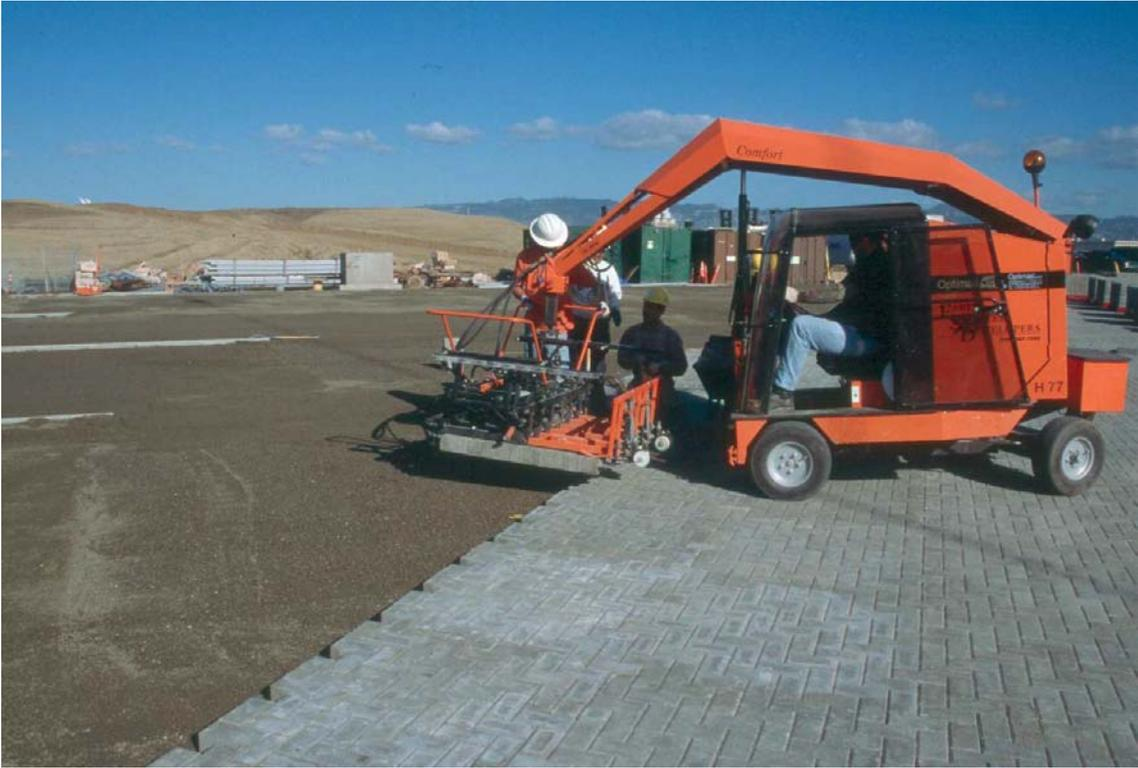
**Figure 4. Mechanized equipment placing interlocking concrete pavement.**
