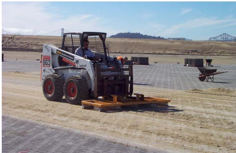
**Figure 9. Spreading joint sand with mounted brooms.**
