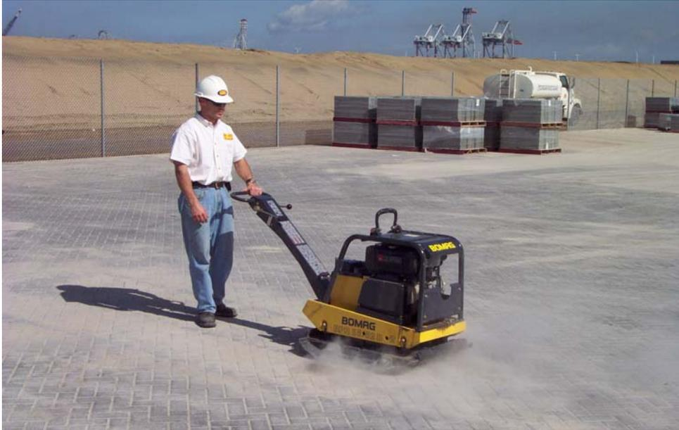
**Figure 10. Final compaction of the pavers with sand swept into the joints.**
