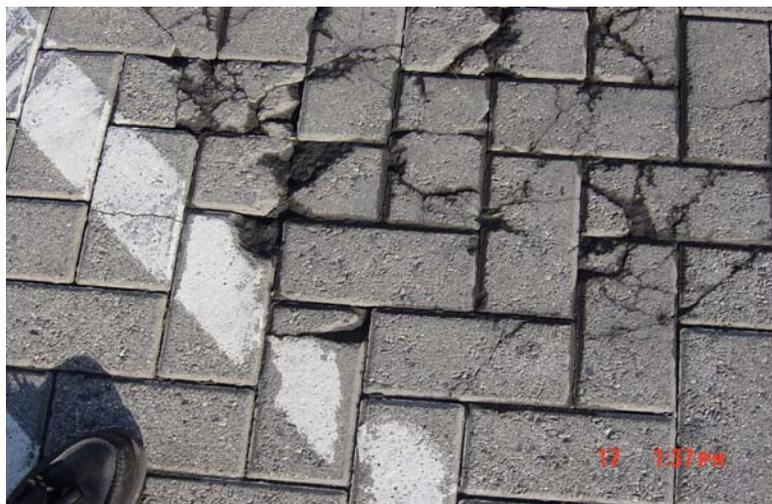
**Figure 1. Showing typical damage under corner castings. This type of damage has caused no loss of service.**
